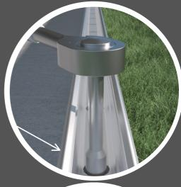
**10.** Place all the clamping plates into the channel
